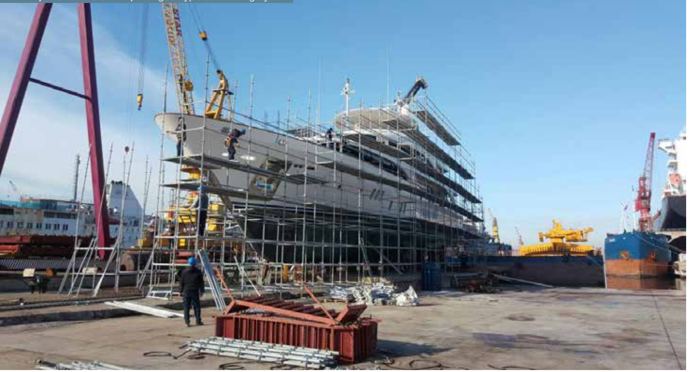
PROJE ADI : KUZEY SHIPYARD YATÇILIK FLANŞLI İSKELE SİSTEMİ / Flanged Type Scaffolding System
