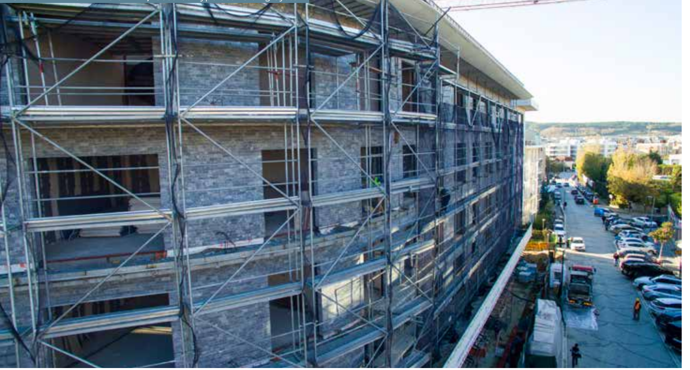
PROJE ADI : LARUS LOFT GÜVENLİKLİ İSKELE SİSTEMİ / Secured Type Scaffolding System
