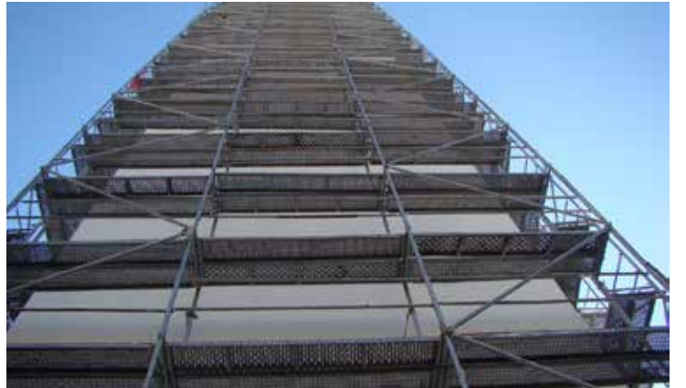
PROJE ADI : NİDAPARK PROJESİ GÜVENLİKLİ İSKELE SİSTEMİ / Secured Type Scaffolding System
